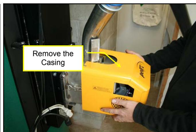
Open the two toggle fasteners, which position the burner body against the mantle's end plate. Angle the burner body and pull it inclined upwards / backwards so that the flame trap pipe releases from the combustion chamber tube.
